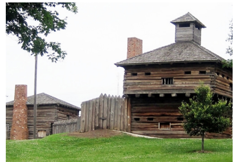
Rebuilt Fort Recovery
